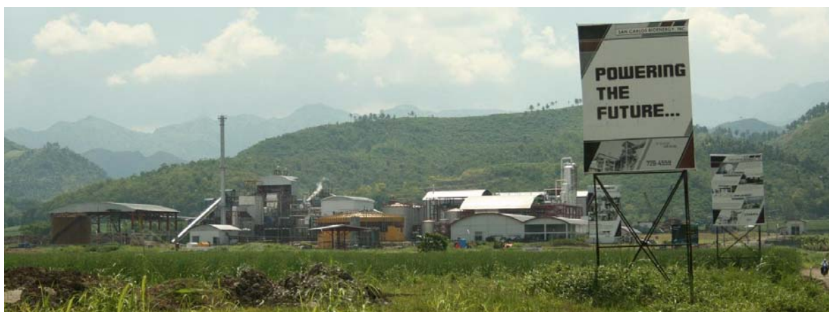
Fig. 1—San Carlos Bio-energy Inc., Philippines ‘Powering the Future’.
