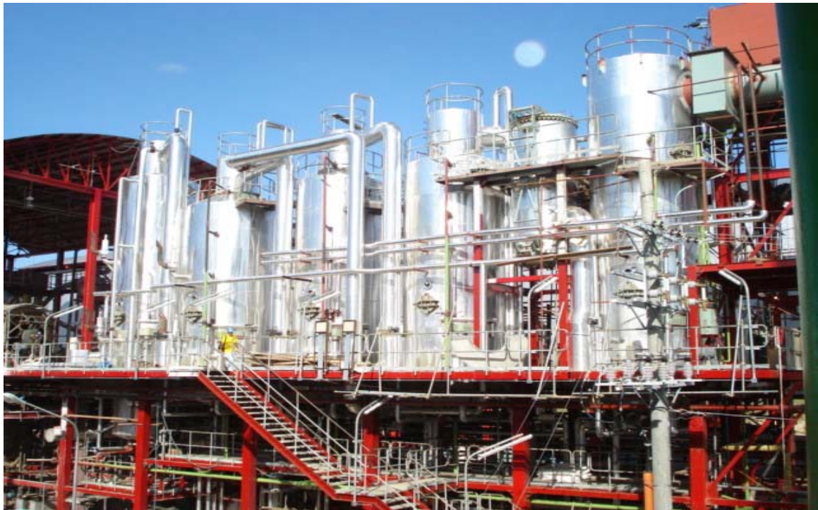
Fig.3—Five effect evaporator set.
