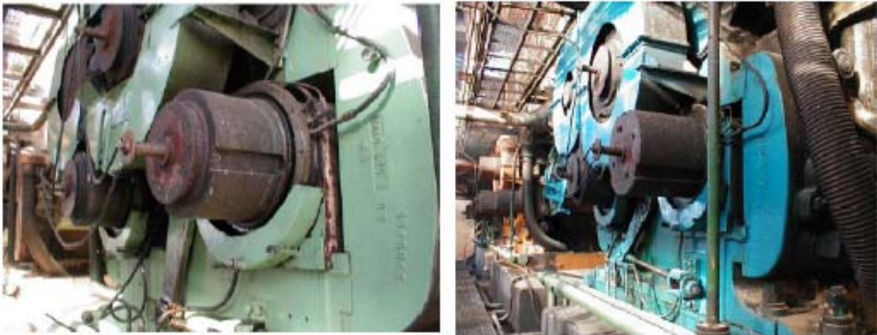
Fig. 6—The absence of spills on the floor prevents accidents.
